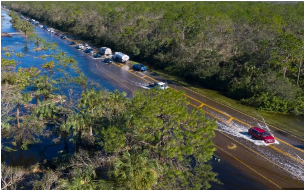
Figure 2-5. Hurricane Ian South River Road Flooding in Sarasota County 51
