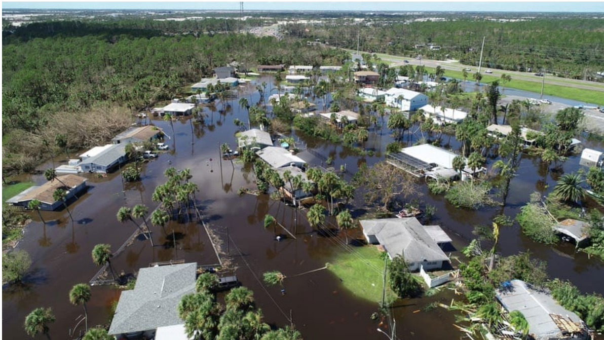
Figure 1-3. Hurricane Ian Damage in City of North Port, Sarasota County 4
