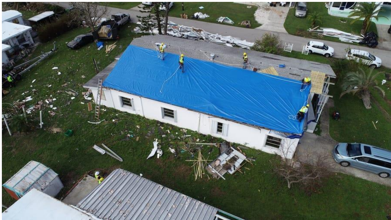
Figure 1-4. Hurricane Ian Housing Damage in Sarasota County 5
