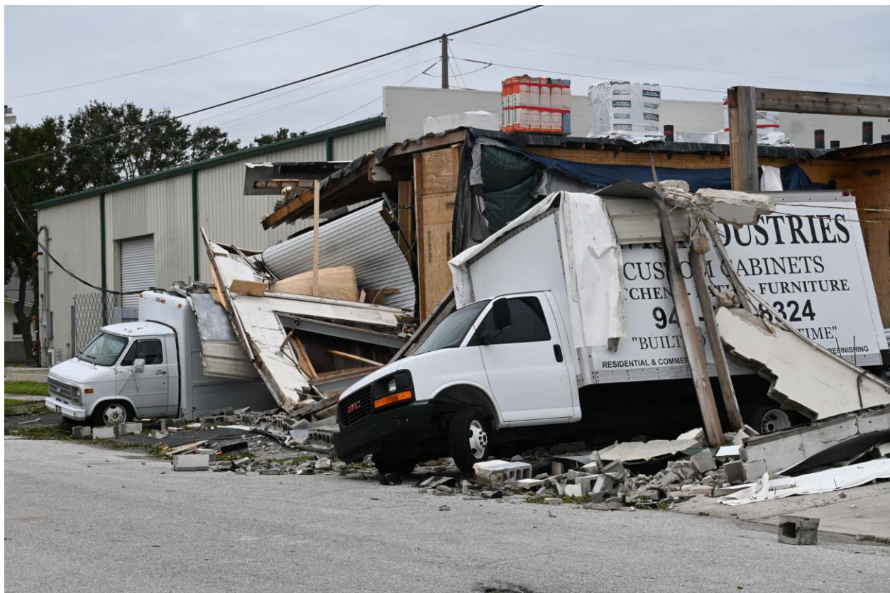
Figure 1-9. Hurricane Damage to Business in Sarasota County 10
