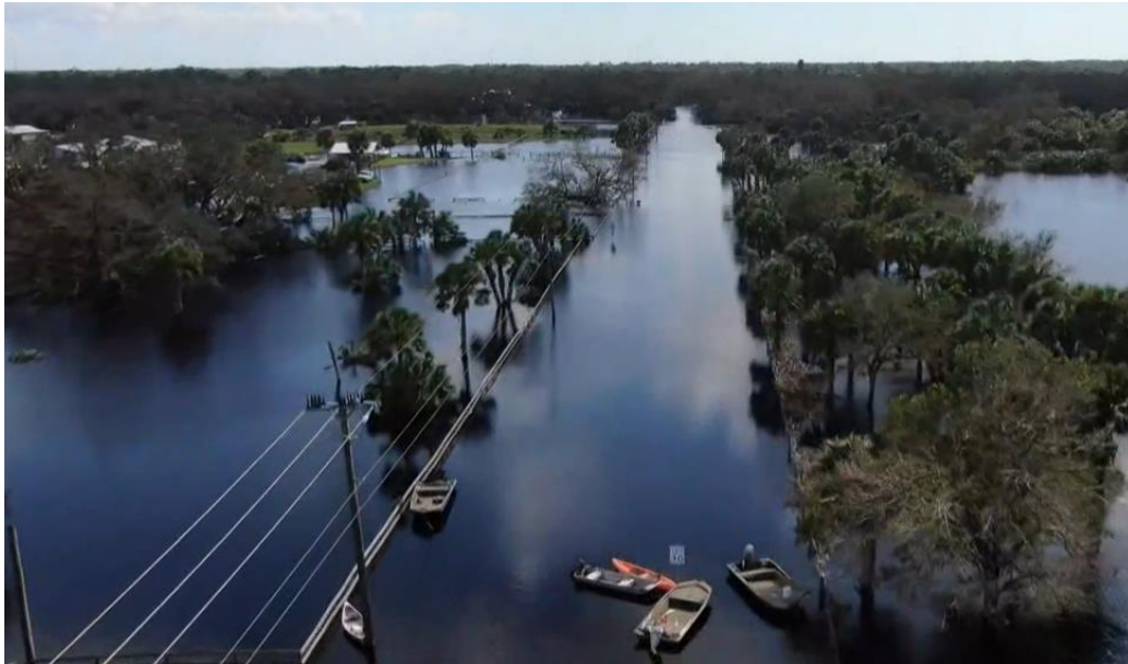
Figure 2-4. Hurricane Ian South River Road Flooding in Sarasota County 50
