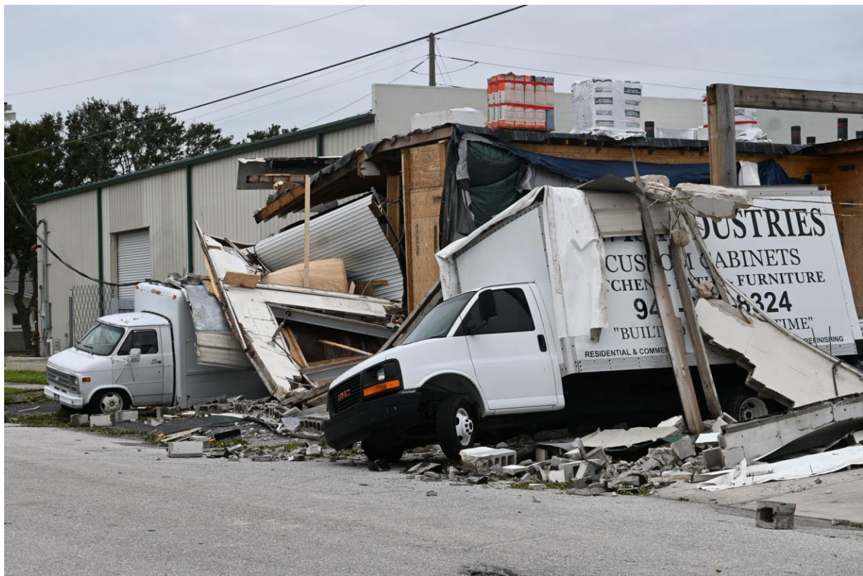
Figure 1-9. Hurricane Damage to Business in Sarasota County 10
