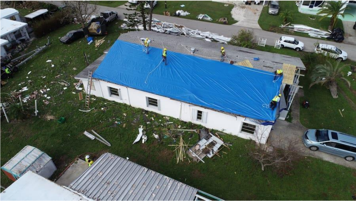
Figure 1-4. Hurricane Ian Housing Damage in Sarasota County 5
