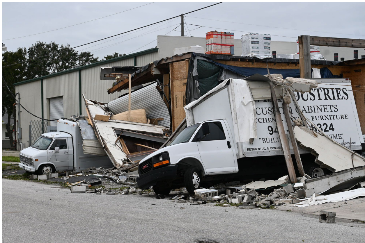
Figure 1-9. Hurricane Damage to Business in Sarasota County 10
