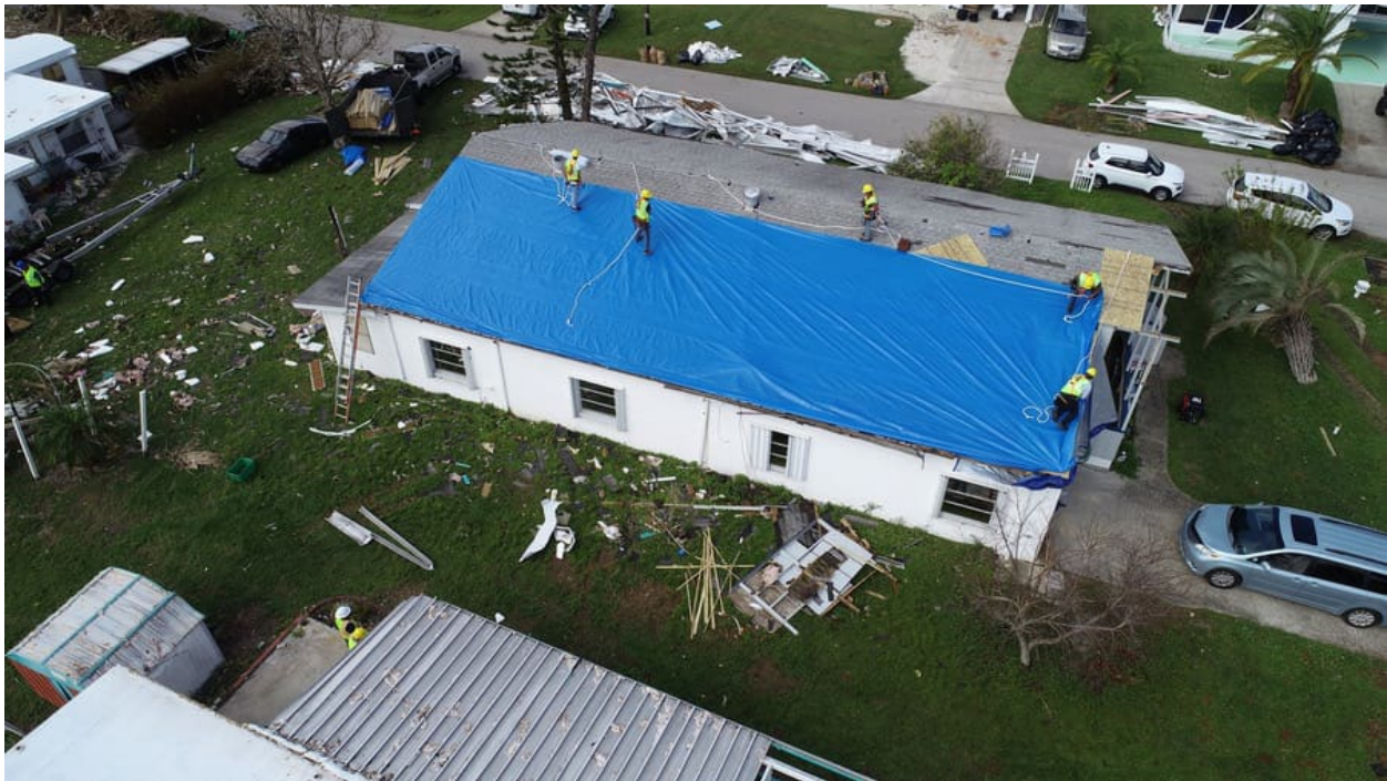
Figure 1-4. Hurricane Ian Housing Damage in Sarasota County 5
