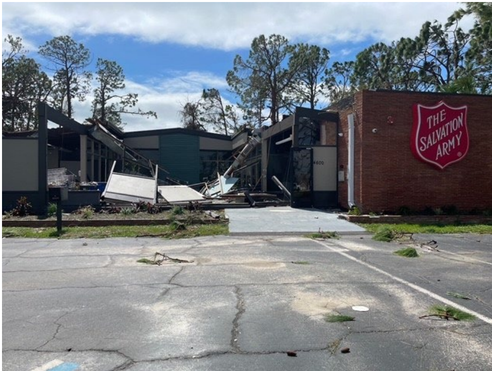
Figure 1-5. Hurricane Ian Damage to the Salvation Army of Sarasota County North Port Facility 6
