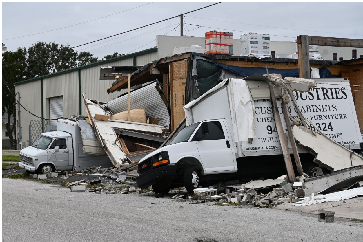
Figure 1-9. Hurricane Damage to Business in Sarasota County 10
