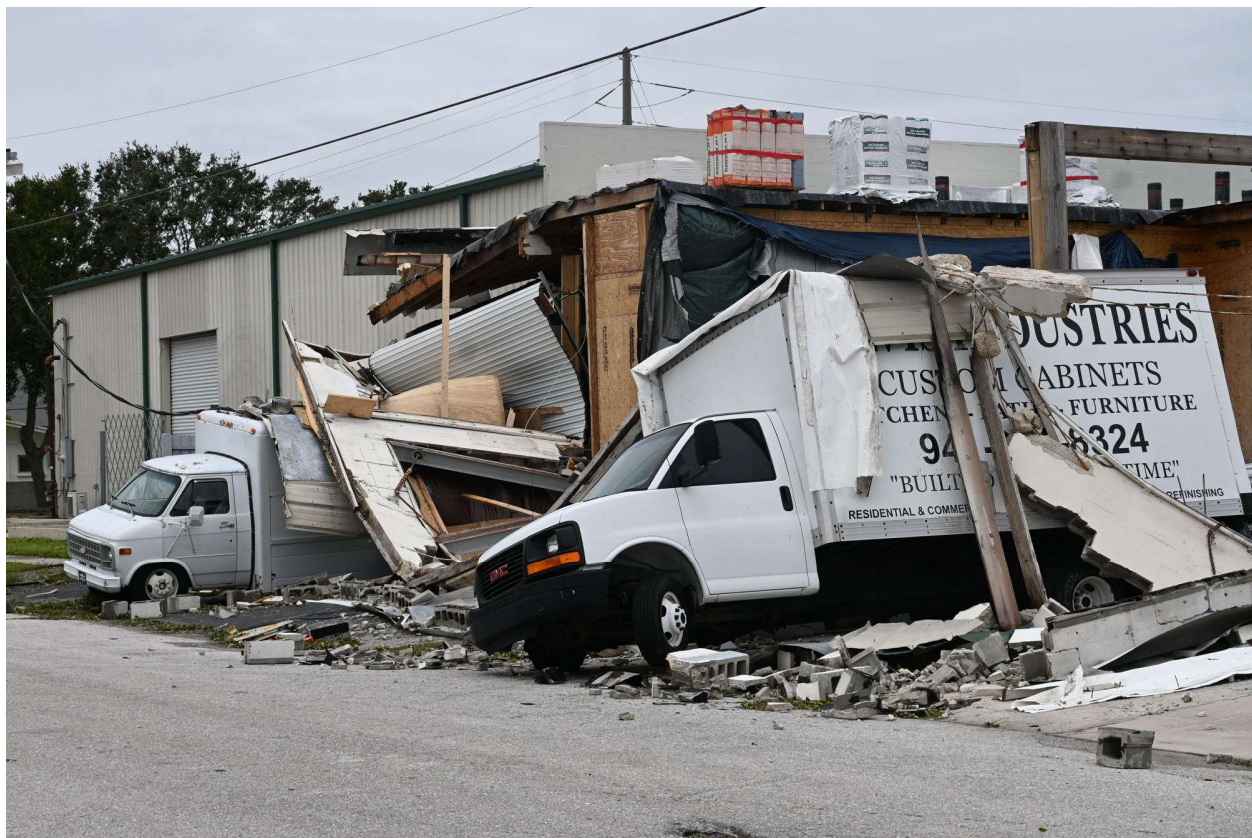
Figure 1-9. Hurricane Damage to Business in Sarasota County 10
